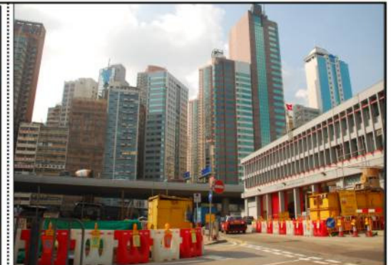
Photo from Baseline Site Visit
