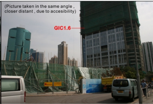
Photo from Baseline Site Visit
