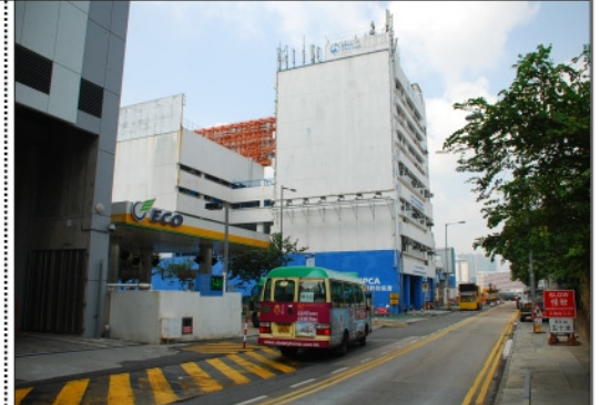
Photo from Baseline Site Visit
