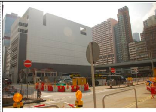
Photo from Baseline Site Visit
