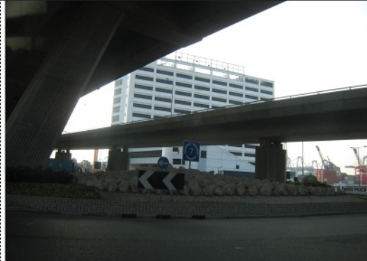
Photo from Baseline Site Visit
