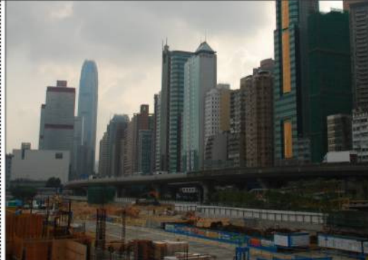
Photo from Baseline Site Visit
