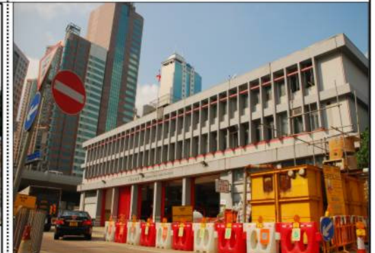
Photo from Baseline Site Visit
