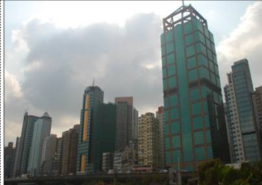
Photo from Baseline Site Visit
