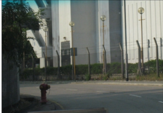
Photo from Baseline Site Visit
