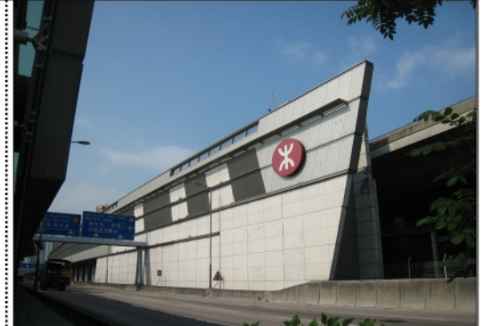
Photo from Baseline Site Visit
