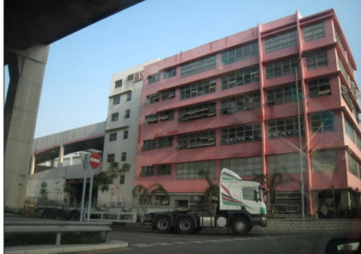
Photo from Baseline Site Visit
