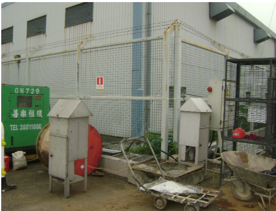
AM6 – Site Boundary at Stonecutters Island Work Site
