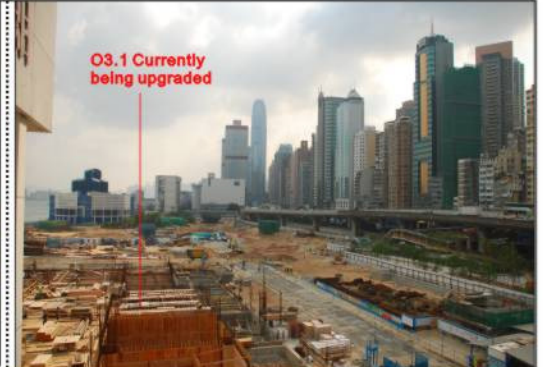
Photo from Baseline Site Visit
