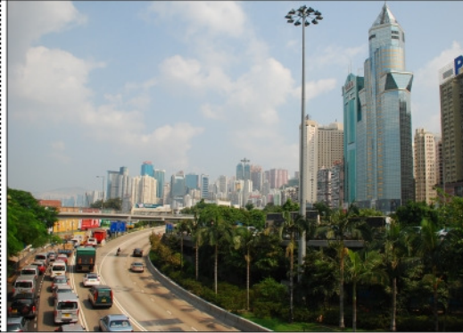
Photo from Baseline Site Visit
