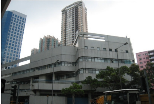
Photo from Baseline Site Visit
