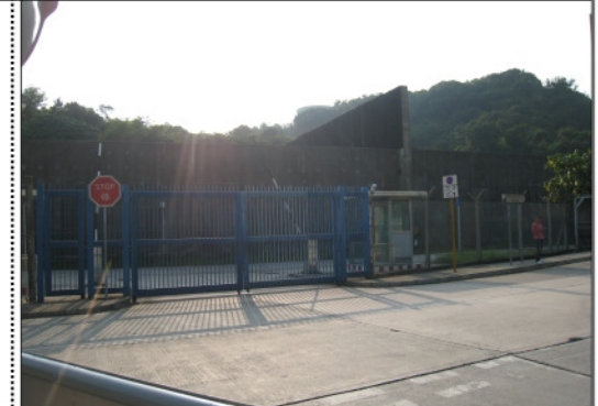
Photo from Baseline Site Visit
