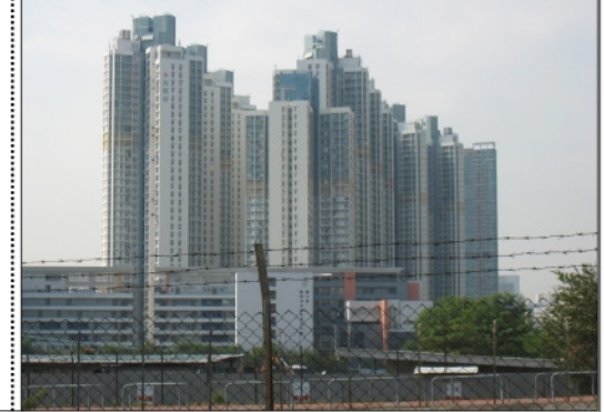
Photo from Baseline Site Visit
