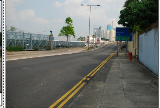
Photo from Baseline Site Visit
