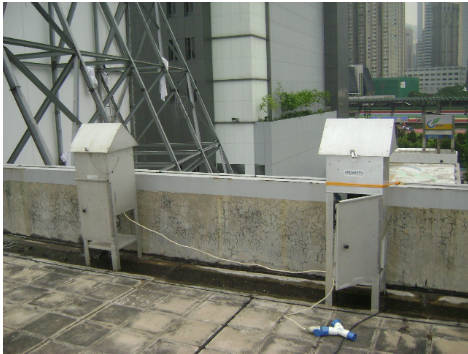
AM3 – Rooftop on DSD Wan Chai East PTW
