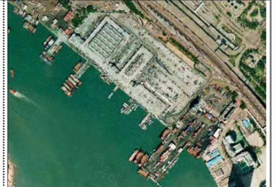
Photo from Baseline Site Visit
