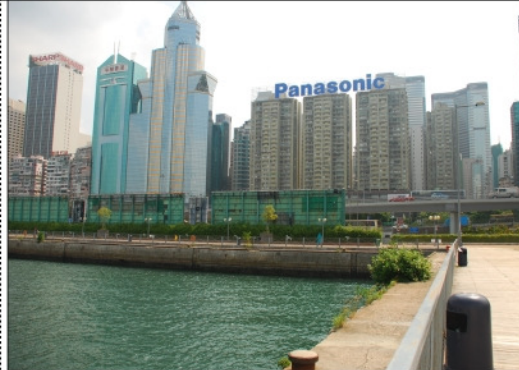
Photo from Baseline Site Visit
