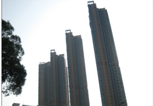
Photo from Baseline Site Visit
