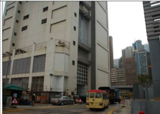
Photo from Baseline Site Visit
