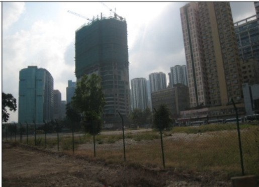
Photo from Baseline Site Visit
