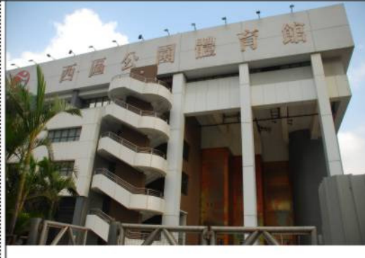
Photo from Baseline Site Visit
