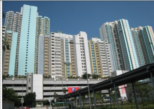
Photo from Baseline Site Visit
