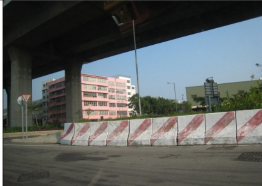
Photo from Baseline Site Visit
