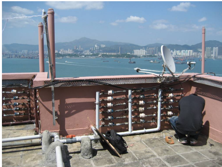
NM4 – Kwan Yick Building Phase III
