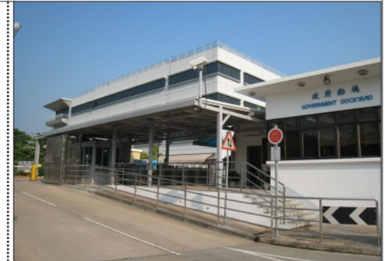
Photo from Baseline Site Visit
